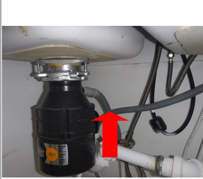
Dishwasher drain line not looped beneath countertop. Recommend repair
