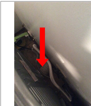
Plastic vent hose not recommended for gas dryer, potential fire hazard.
