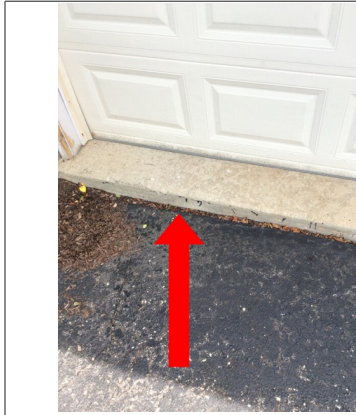
Trip hazard in driveway, recommend repair and/or replacement
