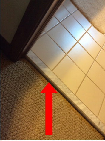
Trip hazard at Bathroom entry, recommend repair/replace transition
