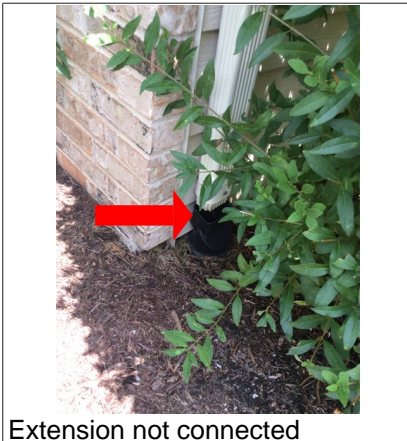
Extension not connected
